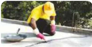
Fill Chemical in Cracks
