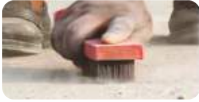
Cleaning by Wire Brush
