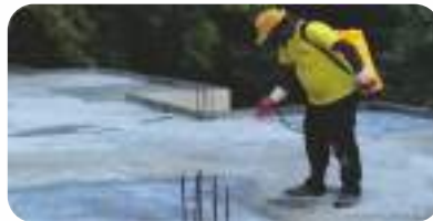
1 st Coat Penetrative Waterproofing
