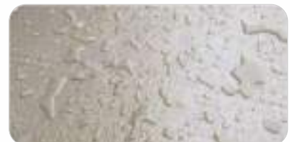
Result After 7 Layer Waterproofing
