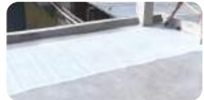
Laying Fibremesh
