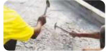
Removing Loose Material
