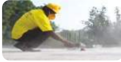
Cleaning by Grinder
